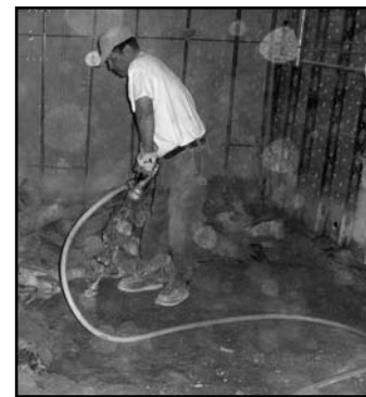
Construction work at Foothill High School
