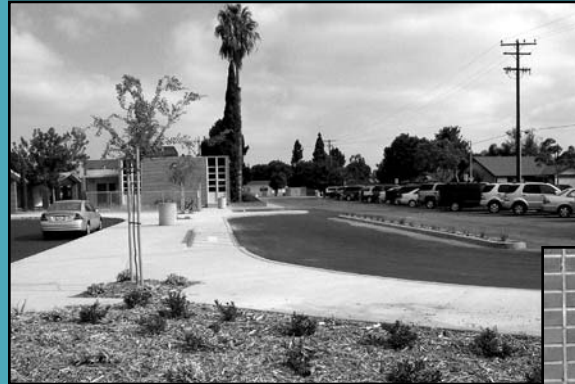
Parking Lot Improvements
