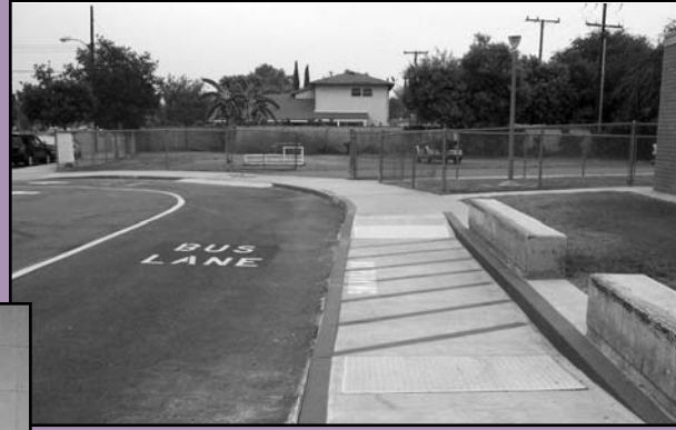
Parking Lot Improvements
