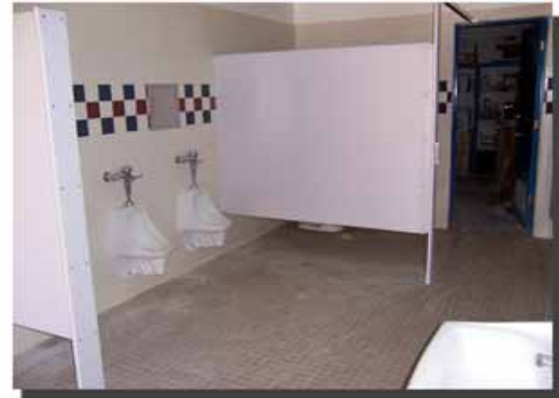
COMPLETED RESTROOM INSTALLATION
