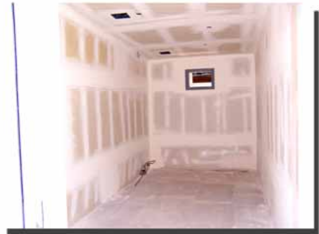
PROGRESS IN ELECTRICAL & JANITORIAL ROOM IN BUILDING "R"
