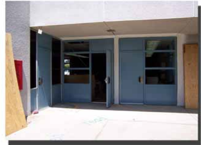
NEW DOORS & WINDOWS INSTALLATION UNDERWAY
