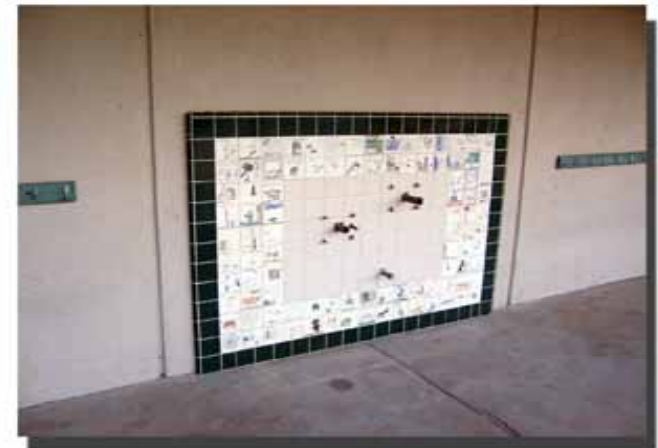
AREA READY FOR NEW OUTDOOR DRINKING FOUNTAIN INSTALLATION
