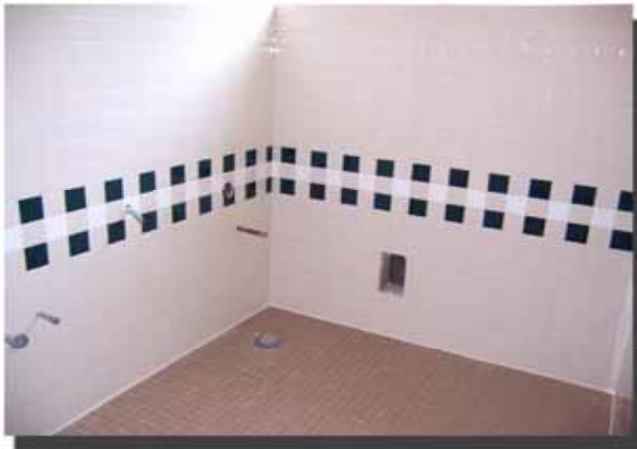
AREA READY FOR NEW SINK & CABINETS FOR THE STUDENT ACTIVITY ROOM
