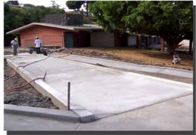
COMPLETED NEW ADA COMPLIANT RAMP
