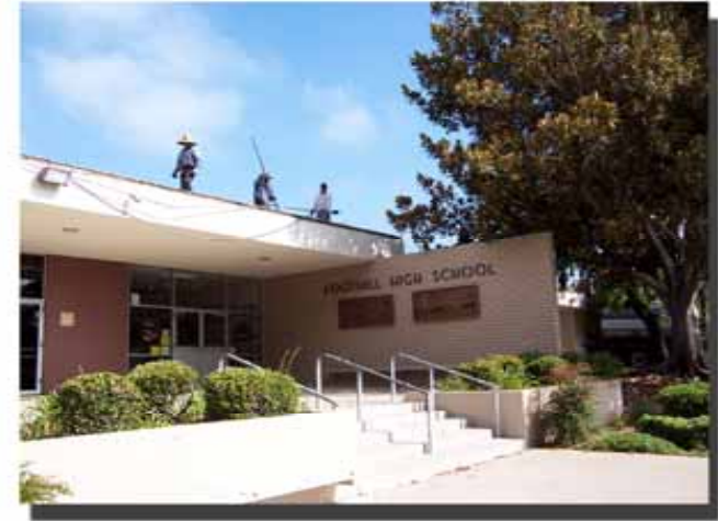
ON-GOING ROOF REPLACEMENT WORK
