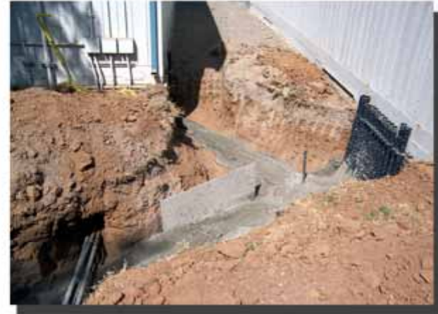
ELECTRICAL CONDUIT TRENCH READY FOR BACKFILL
