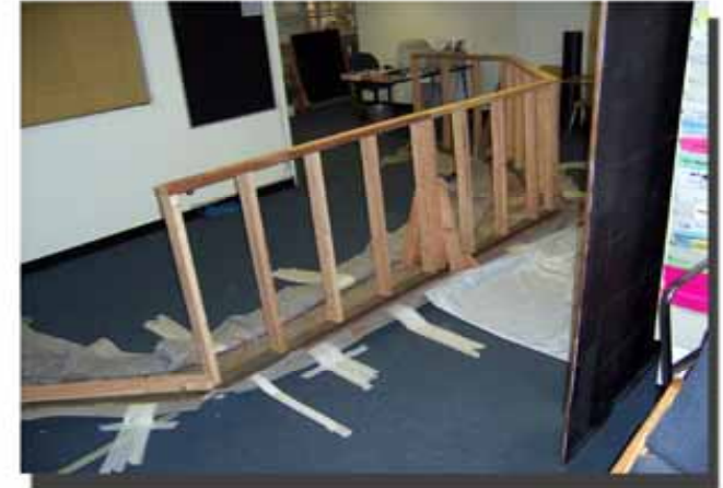
ATTENDANCE ROOM AREA READY FOR NEW CASEWORK INSTALLATION
