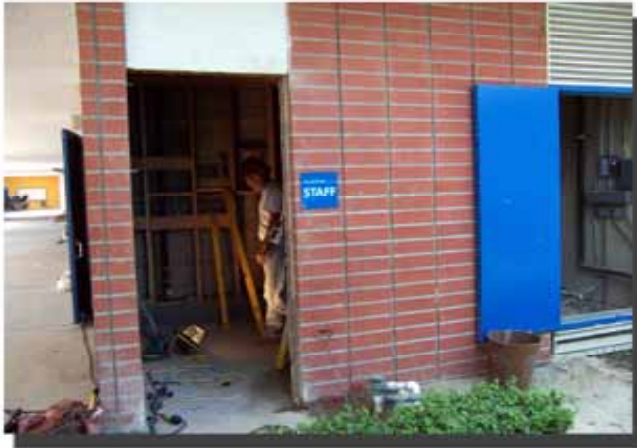
ROUGH PLUMBING WORK & FRAMING UNDERWAY AT STAFF RR IN ADMINISTRATION BLDG.
