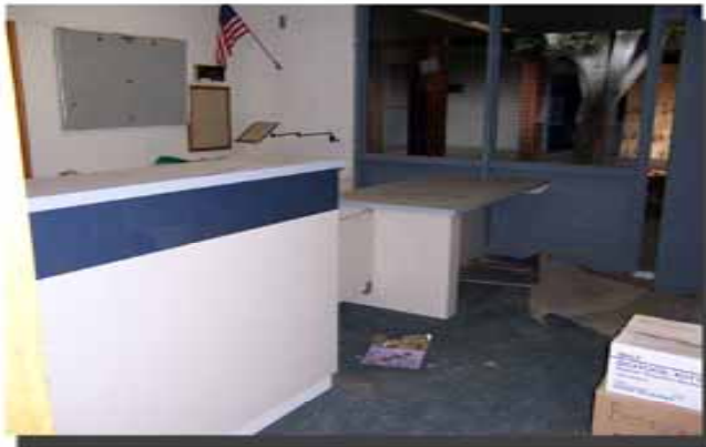
COMPLETED DOOR / WINDOW ASSEMBLY & ADA COMPLIANT COUNTERTOP AT ADMINISTRATION BUILDING
