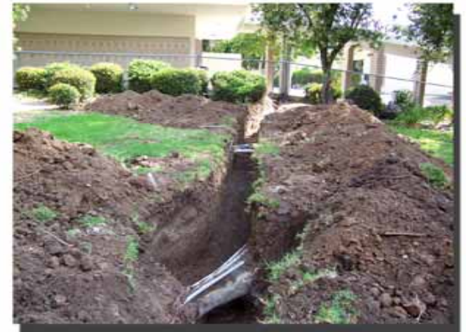
TRENCH WORK IN PROGRESS FOR ELECTRICAL CONDUITS
