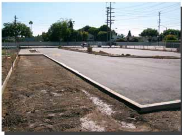
PAVED PARENTS' DROP-OFF AREA WITH SIDEWALK READY FOR CONCRETE POUR
