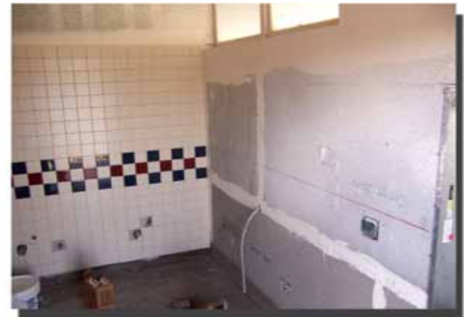
PROGRESS OF RESTROOM MODERNIZATION WORK - TILE INSTALLATION UNDERWAY
