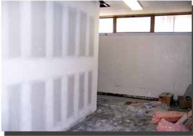
MODIFIED REST AREA IN ADMINISTRATION BUILDING
