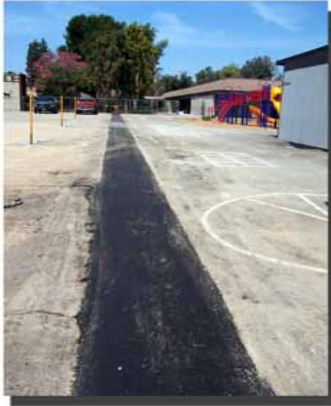
COMPLETED ELECTRICAL TRENCH WORK
