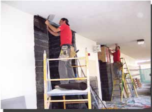
EXTERIOR WORK FOR RESTROOMS ACCESS
