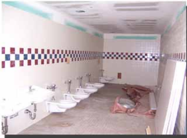
NEW RESTROOM READY FOR CEILING PAINTING & STALL PARTITIONS INSTALLATION
