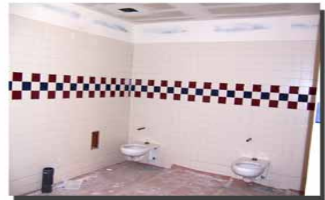
RESTROOM INSTALLATION READY FOR CEILING PAINTING, LIGHT FIXTURES, & PARTITIONS
