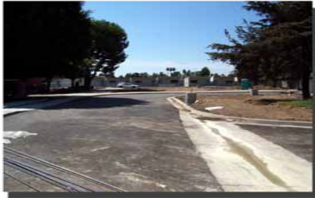
BUS DROP-OFF DRIVEWAY NEAR COMPLETION
