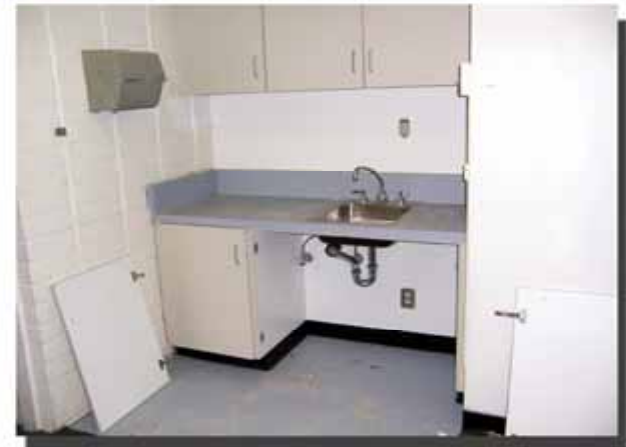
NEW SINK INSTALLATION IN ADMINISTRATION BUILDING
