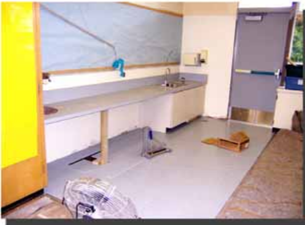
NEAR-COMPLETION SINK & COUNTERTOP INSTALLATION IN CLASSROOM
