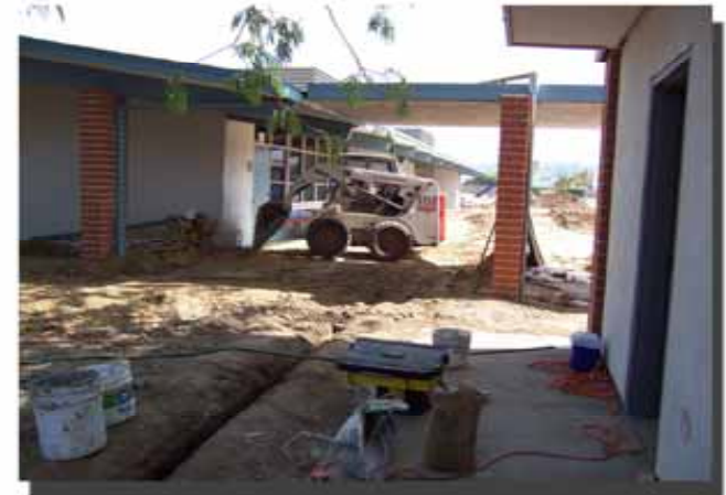
ELECTRICAL TRENCH BACKFILLING & SITE CLEAN-UP ACTIVITIES
