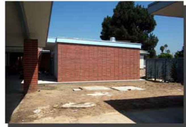
NEAR-COMPLETION STAFF RESTROOM BUILDING
