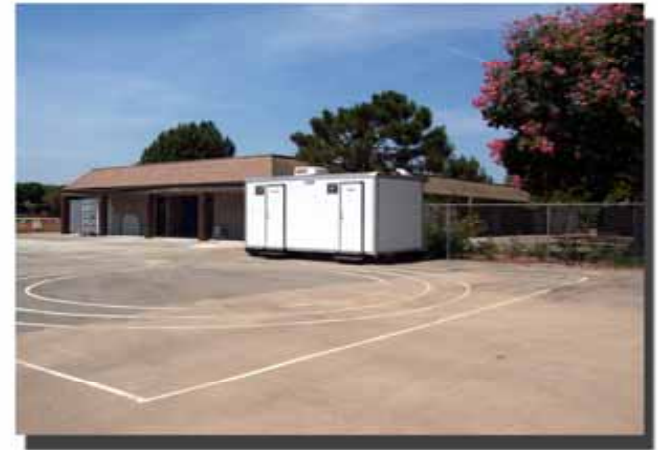
TEMPORARY RESTROOM INSTALLATION FOR STUDENTS READY ON SITE
