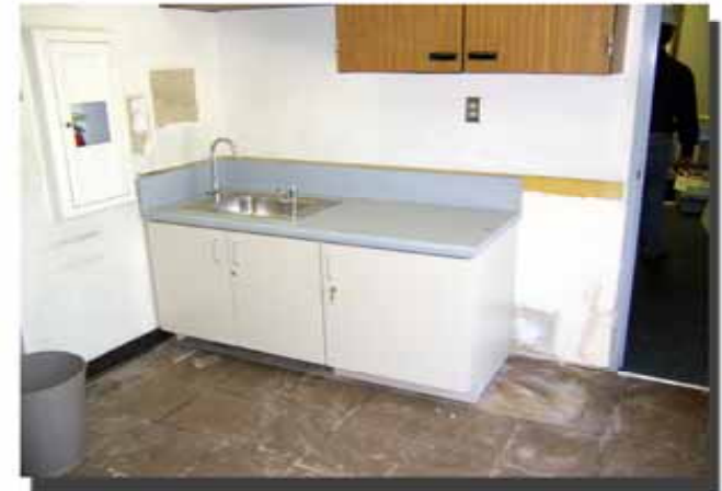
WORK IN PROGRESS - INSTALLATION OF ADA COMPLIANT CABINET WITH SINK
