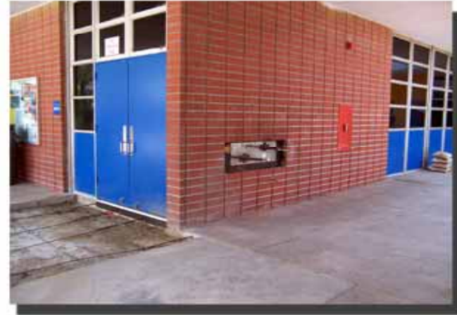
PROGRESS WORK FOR ADA COMPLIANT EXIT WAY RAMP & DRINKING FOUNTAIN
