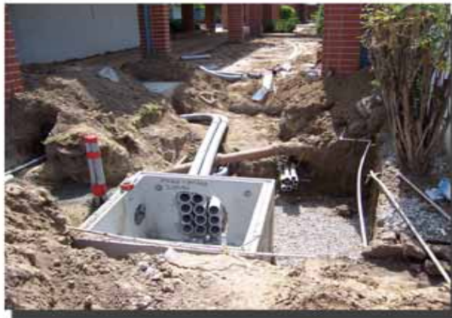
INSTALLATION OF UNDERGROUND FIRE ALARM CONDUITS & ELECTRICAL VAULT
