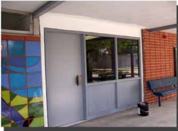
COMPLETED EXTERIOR DOOR & WINDOWS IN ADMINISTRATION BUILDING
