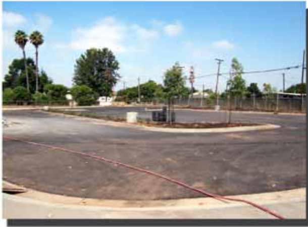
COMPLETED PARKING LOT PAVING & IN-PROGRESS LANDSCAPE INSTALLATION
