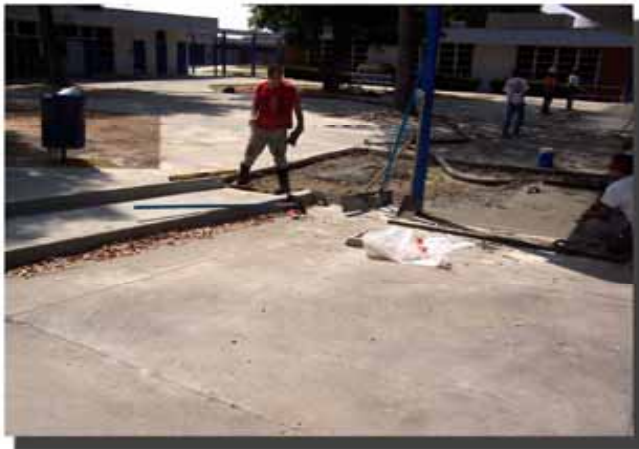
COMPLETION OF ADA COMPLIANT RAMP & WALKWAY
