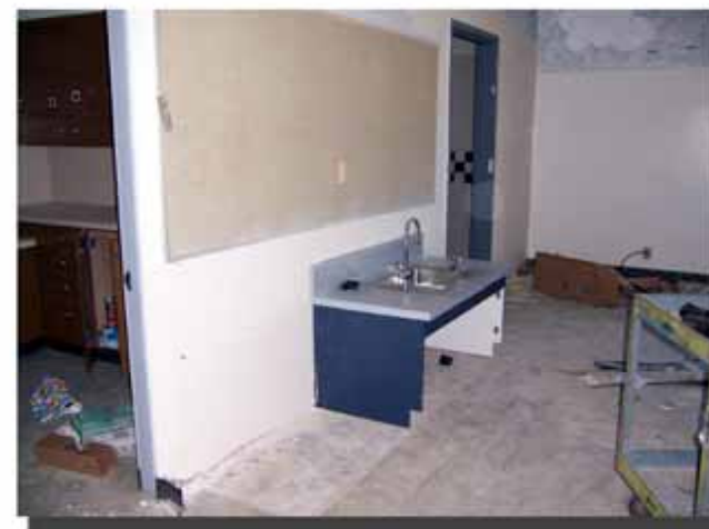
NEW SINK INSTALLATION IN THE KINDERGARTEN AREA
