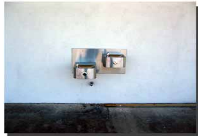
COMPLETED OUTDOOR DRINKING FOUNTAIN
