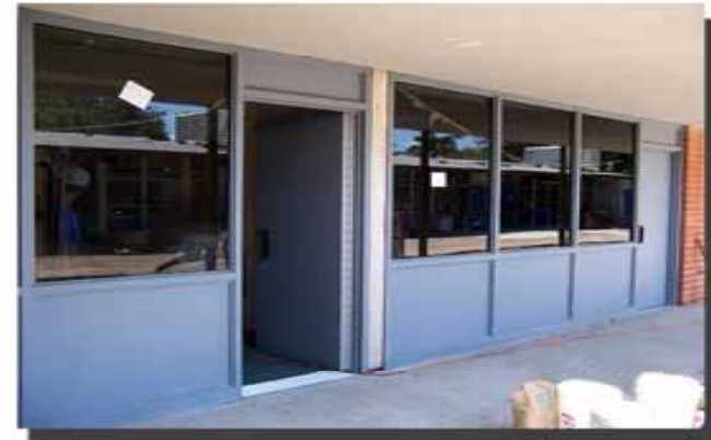
NEW WINDOW FRONT, DOOR, & SIDEWALK INSTALLATION FOR ADMINISTRATION BUILDING
