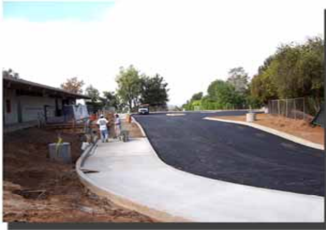
COMPLETED PARKING PAVING & IN-PROGRESS PEDESTRIAN RAMP WORK
