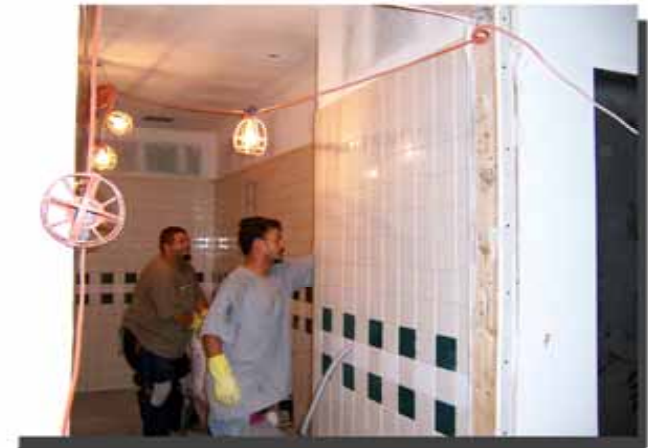
WORK FOR STAFF RESTROOMS IN ADMINISTRATION BUILDING
