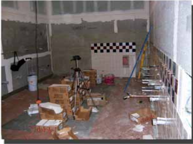
RESTROOM WORK PROGRESS: ROUGH PLUMBING IN PLACE & START OF TILE INSTALLATION
