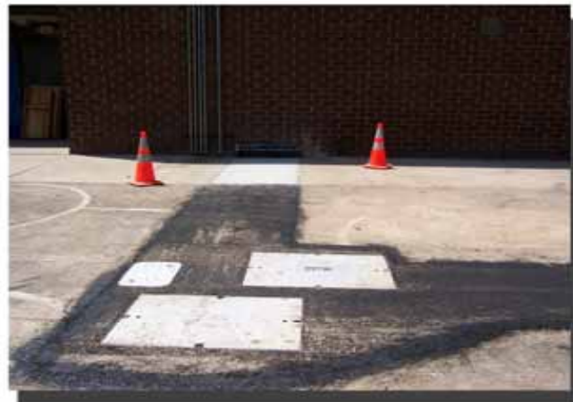
COMPLETED UNDERGROUND ELECTRICAL VAULTS & CONDUITS INSTALLATION
