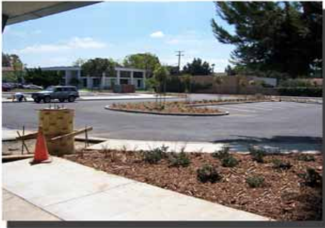
NEW PARKING LOT READY FOR NEW LIGHT POLES
