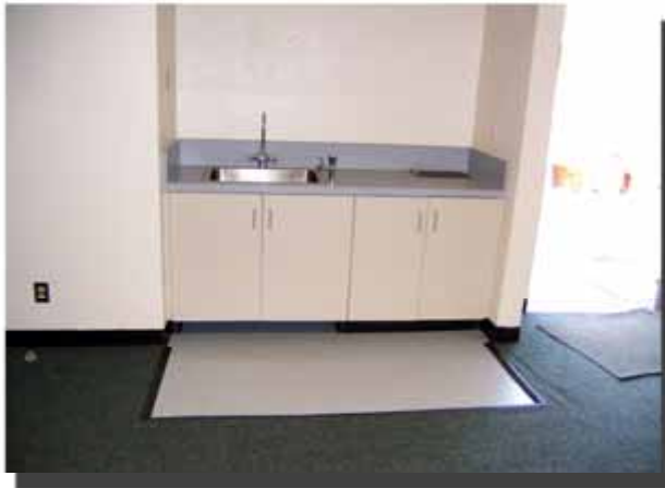
COMPLETED ADA COMPLIANT SINK, CABINETS, & NEW VINYL FLOORING
