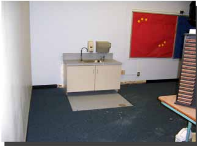
NEW CABINET & SINK NEAR COMPLETION
