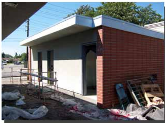
STAFF RESTROOM & ELECTRICAL ROOM BUILDING WORK
